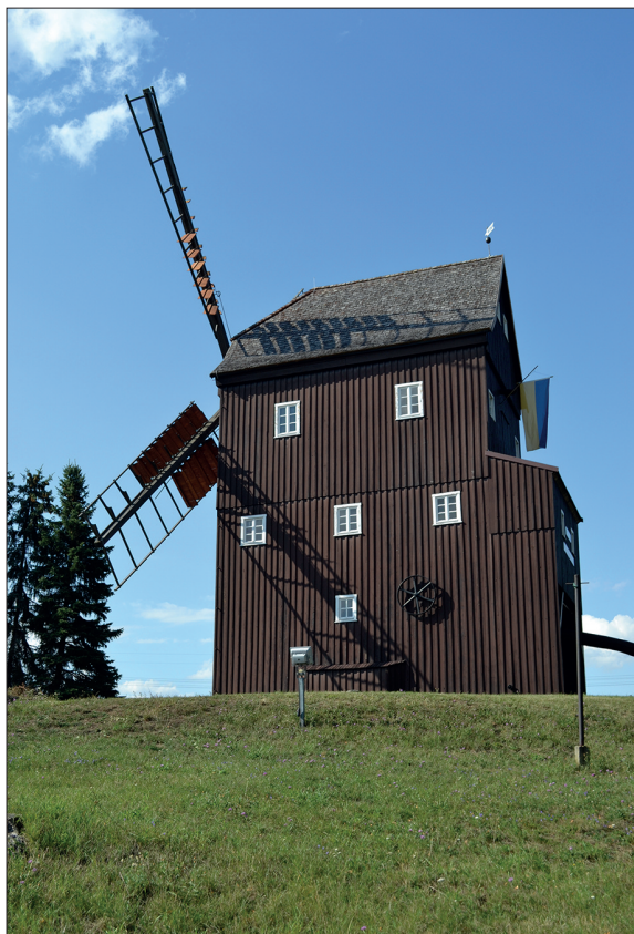
Fig. 11. Neumann Mühle, a post mill 'retro-fitted' as a paltrok mill (G. Hackney).
