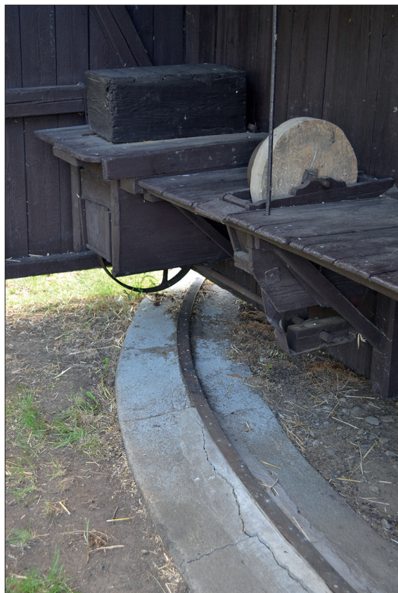
Fig. 12. Neumann Mühle, the rail for the four supporting wheels (G. Hackney).
